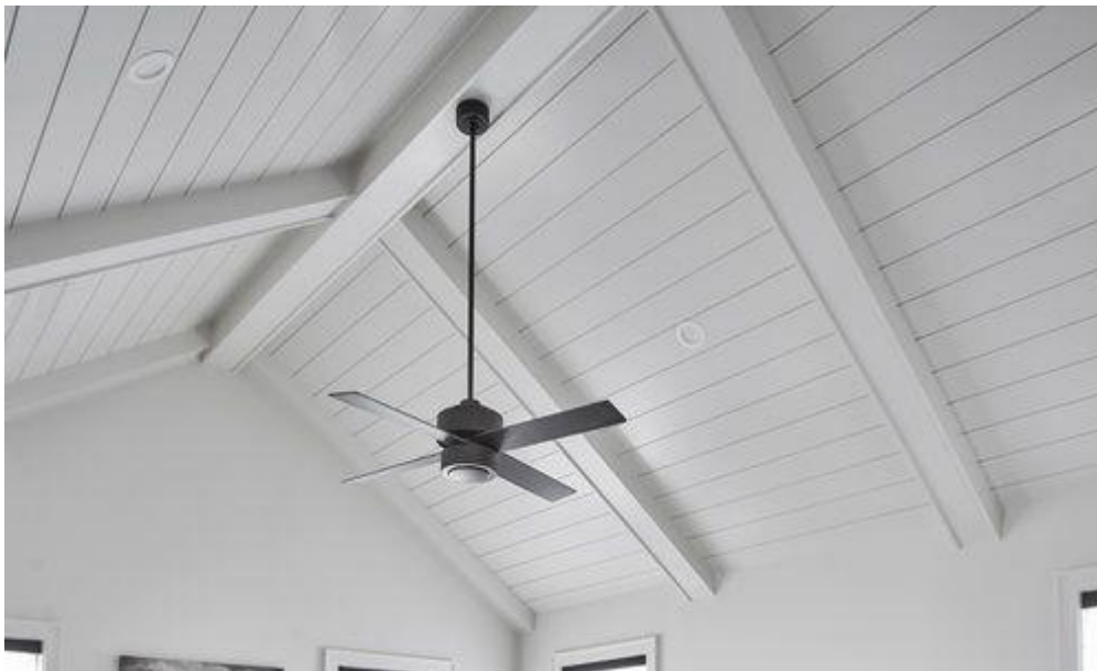
OWNERS BEDROOM CEILING BEAMS & SHIPLAP
