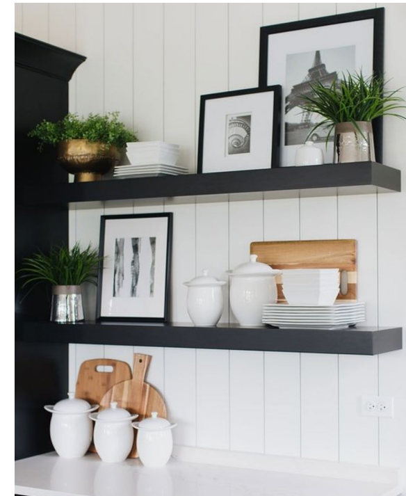
8" PLANK VERTICAL SHIPLAP FROM COUNTERTOP TO CEILING
