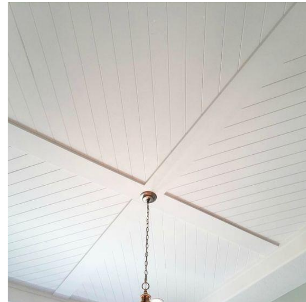
OWNERS BEDROOM CEILING DETAIL
