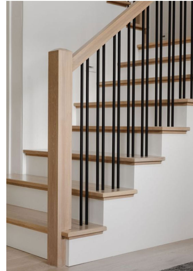
WROUGHT IRON STAIR BALUSTERS, SQUARE NOSINGS AND WOOD CHAMFER NEWELS
