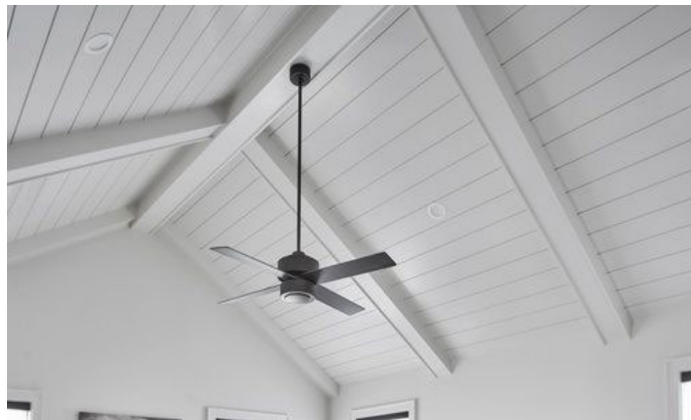
OWNERS BEDROOM CEILING BEAMS & SHIPLAP
