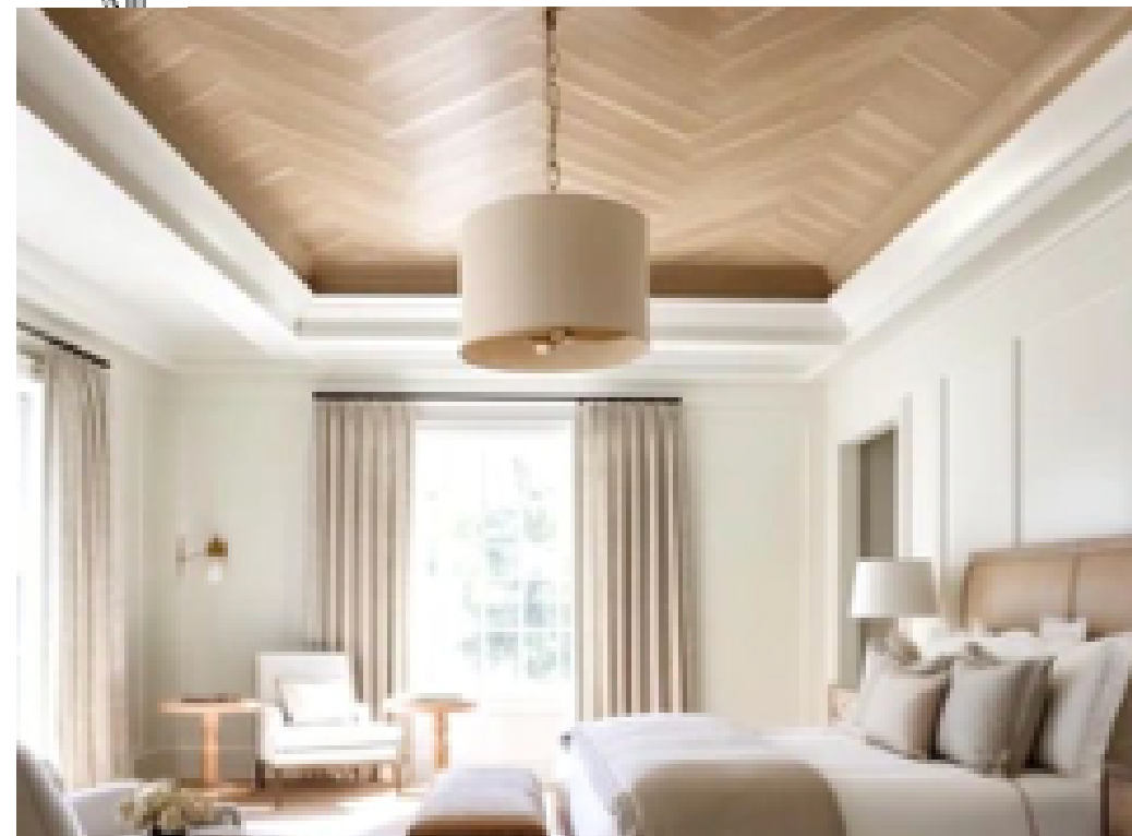
OWNERS SUITE | TRAY CEILING DETIAL WITH A 1 BY 6 HERRINGBONE WHITE OAK DETAIL (STAINED)
